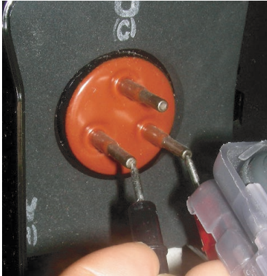
* Measuring resistance between each terminal of compressor
